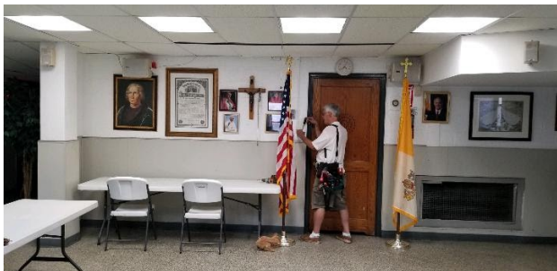
Bro. Joe Saccente finishing new lighting installation in the Cafeteria.
